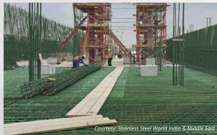
The interior of one of the reservoirs under construction. A green Fusion Bonded Epoxy (FBE) coating protects the steel reinforcing bar against corrosion. © Big Blue Trading and Contracting
